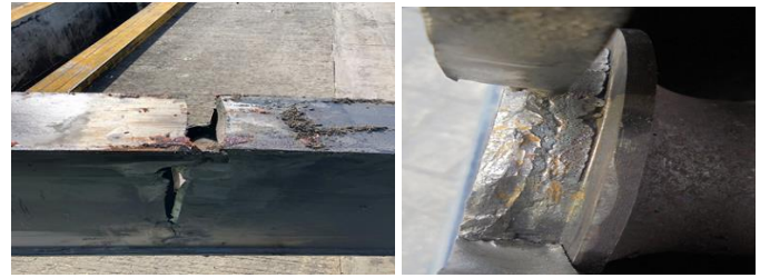
Fig 7. Welding between cylindrical separator and sheet.
