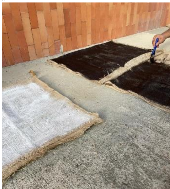
Fig. 5. Coating application process
