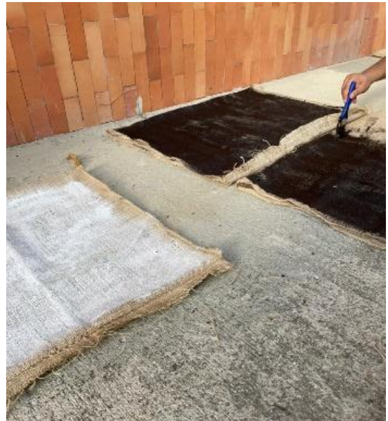
Fig. 5. Coating application process
