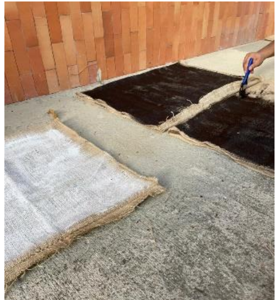
Fig. 5. Coating application process
